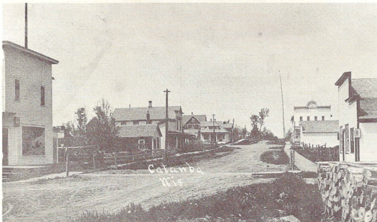
View looking north from R.R. tracks.
