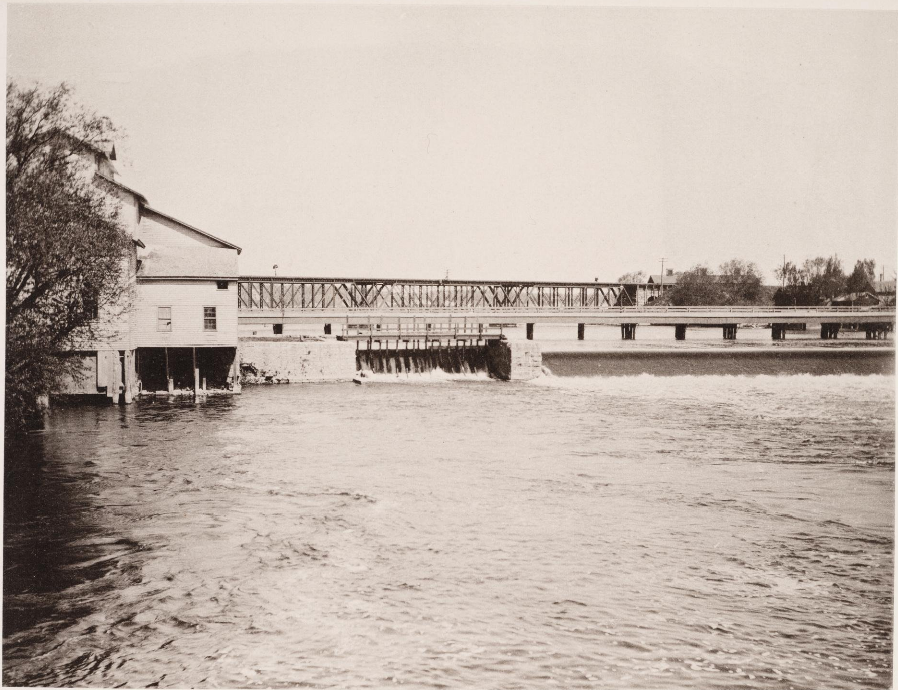
UPPER DAM AT JANESVILLE.
