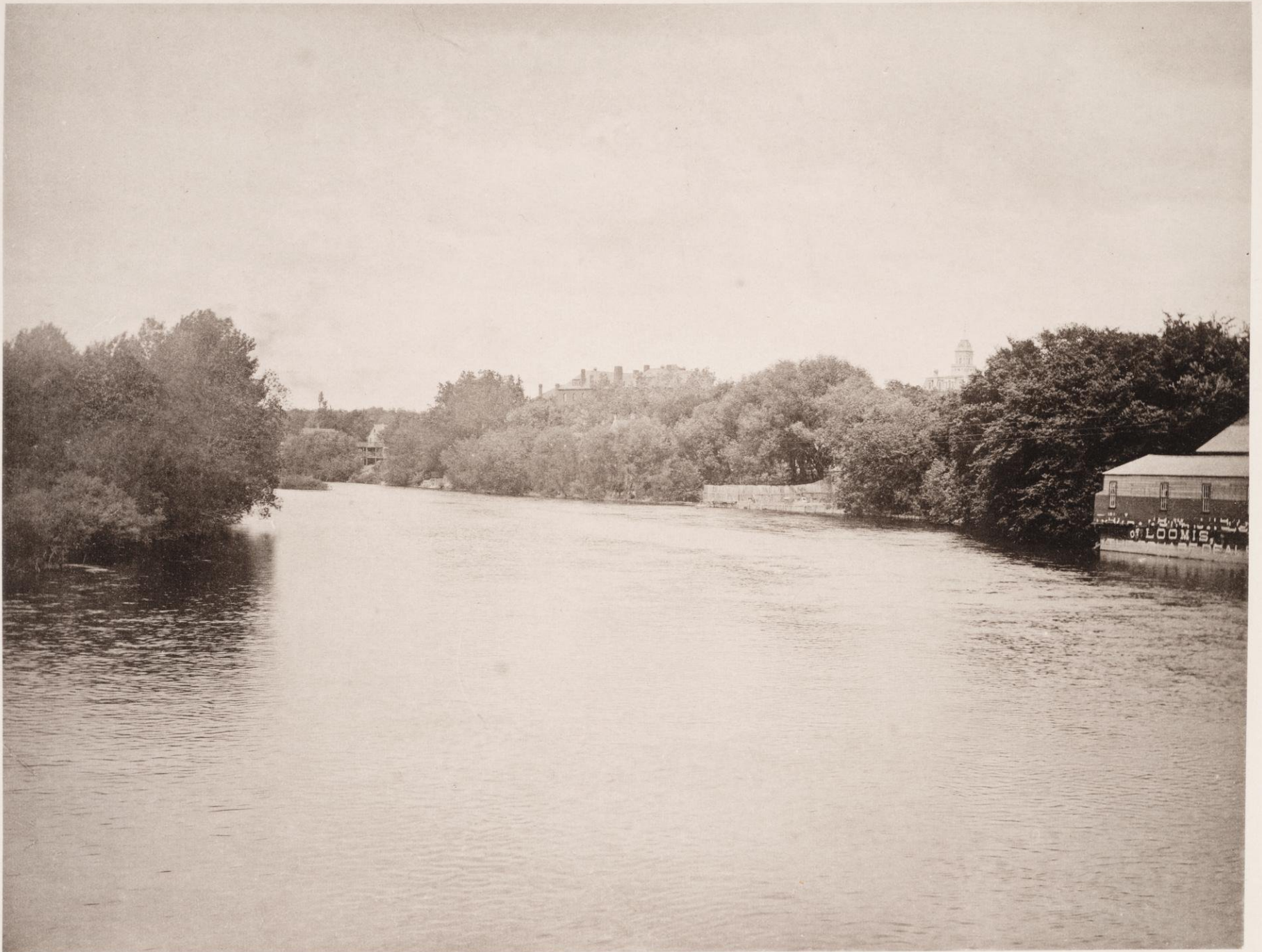
LOOKING NORTH FROM BRIDGE—BELOIT.
