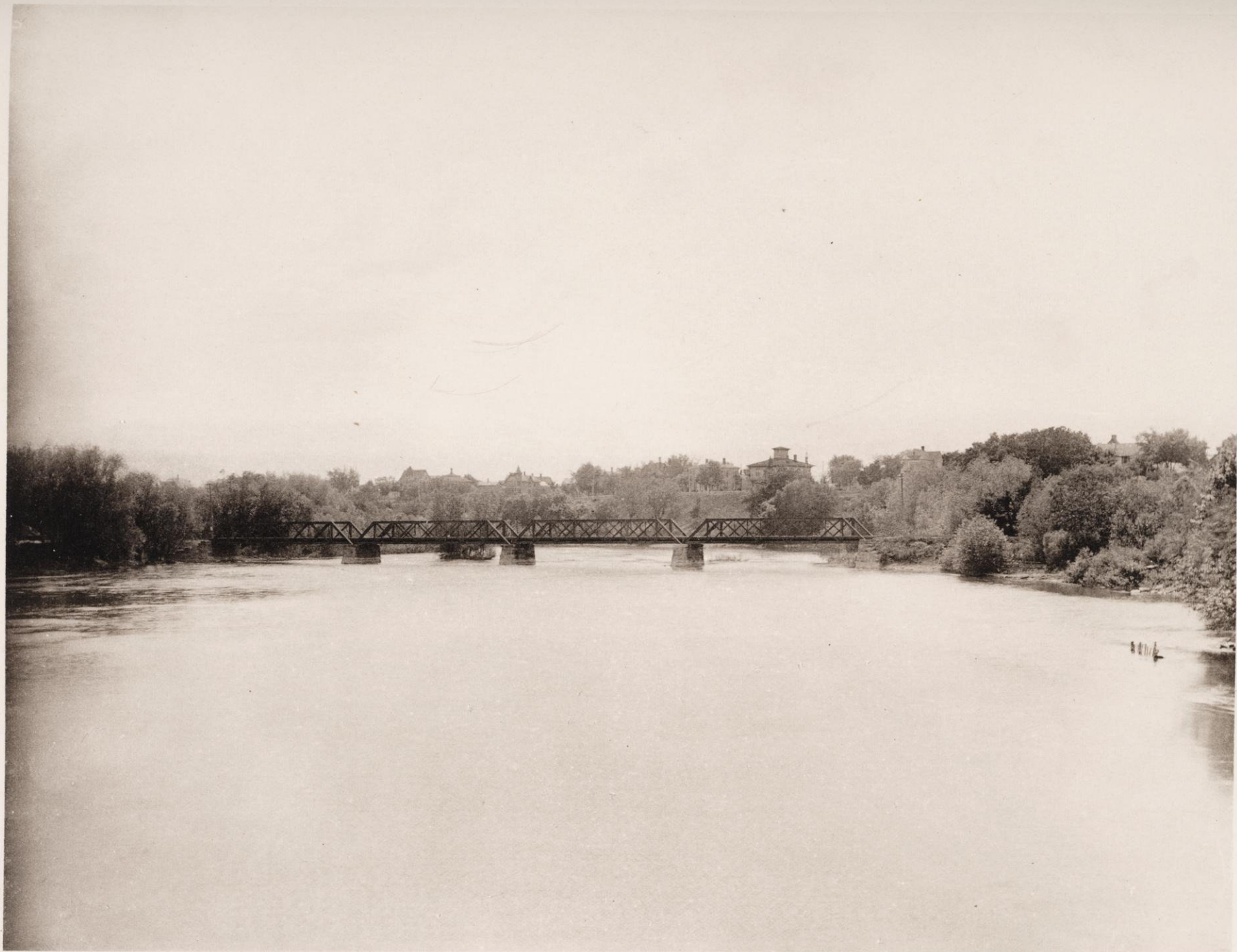
LOOKING SOUTHWEST FROM BRIDGE—BELOIT.
