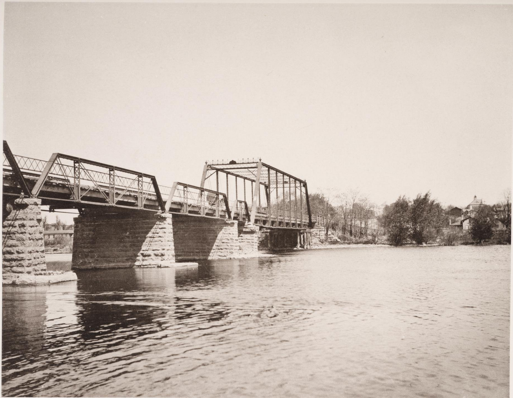
MONTEREY ROAD BRIDGE.
