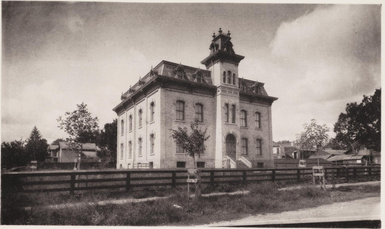
Central School Building.
