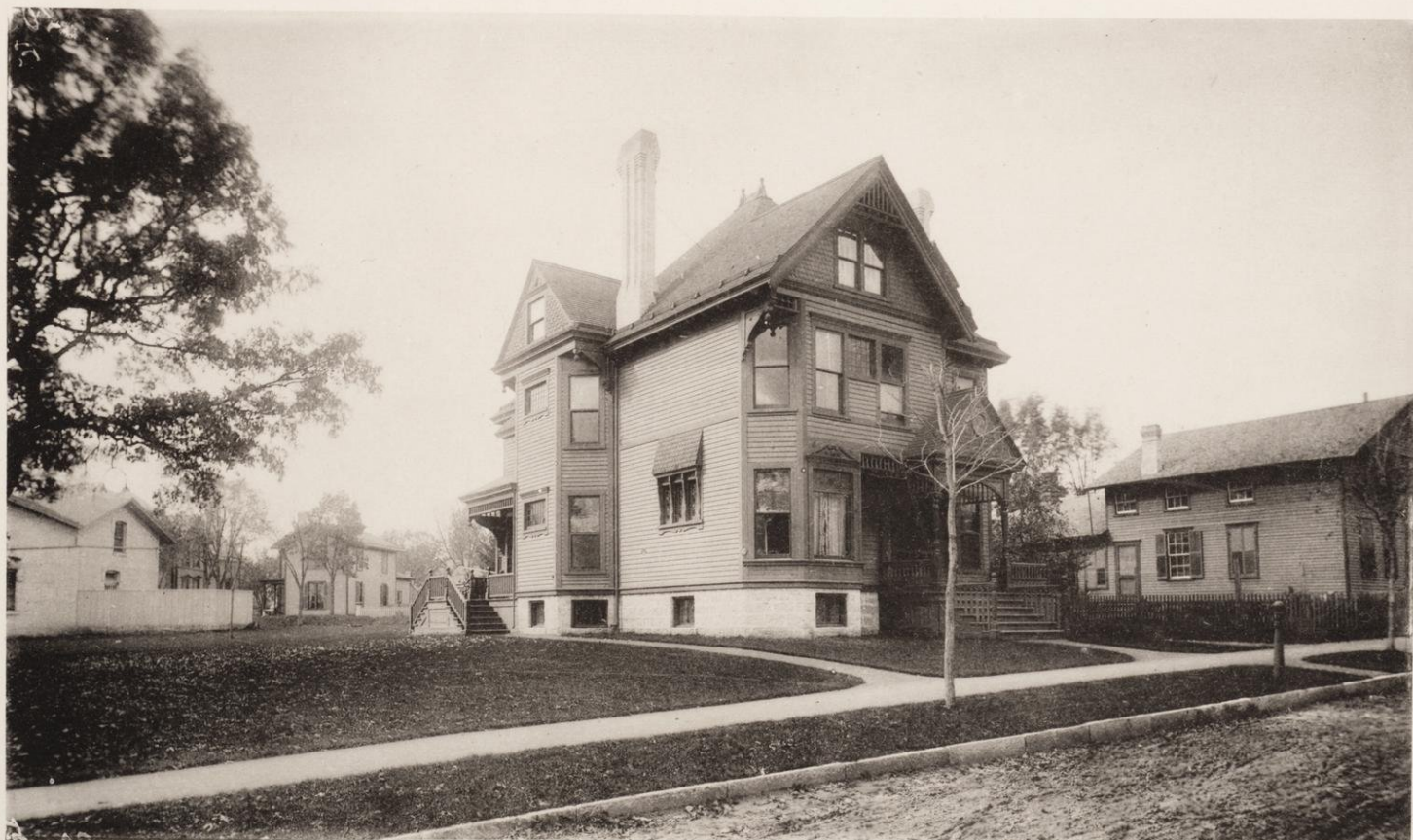
Residence of Leod H. Becker.
