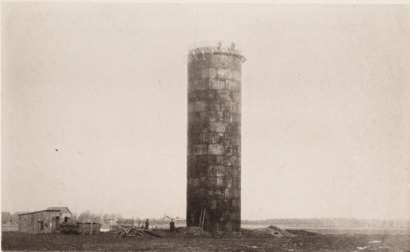
Stand Pipe of Water Works.
