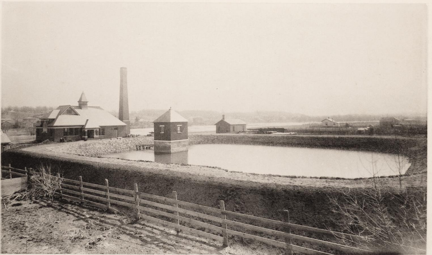
Reservoir and Engine House, Janesville Water Works.
