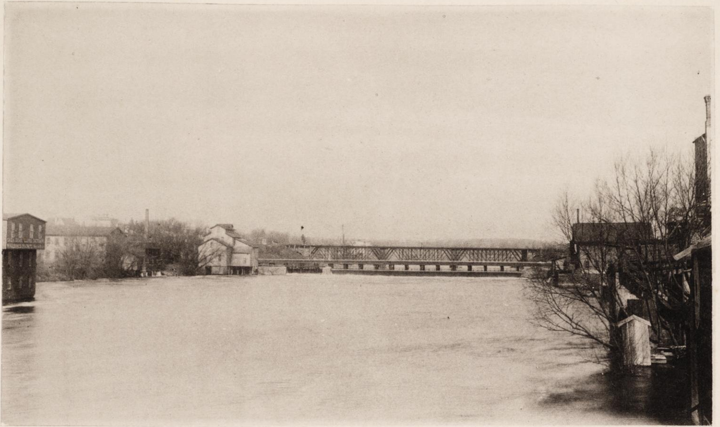
Up River from Milwaukee Street Bridge.
