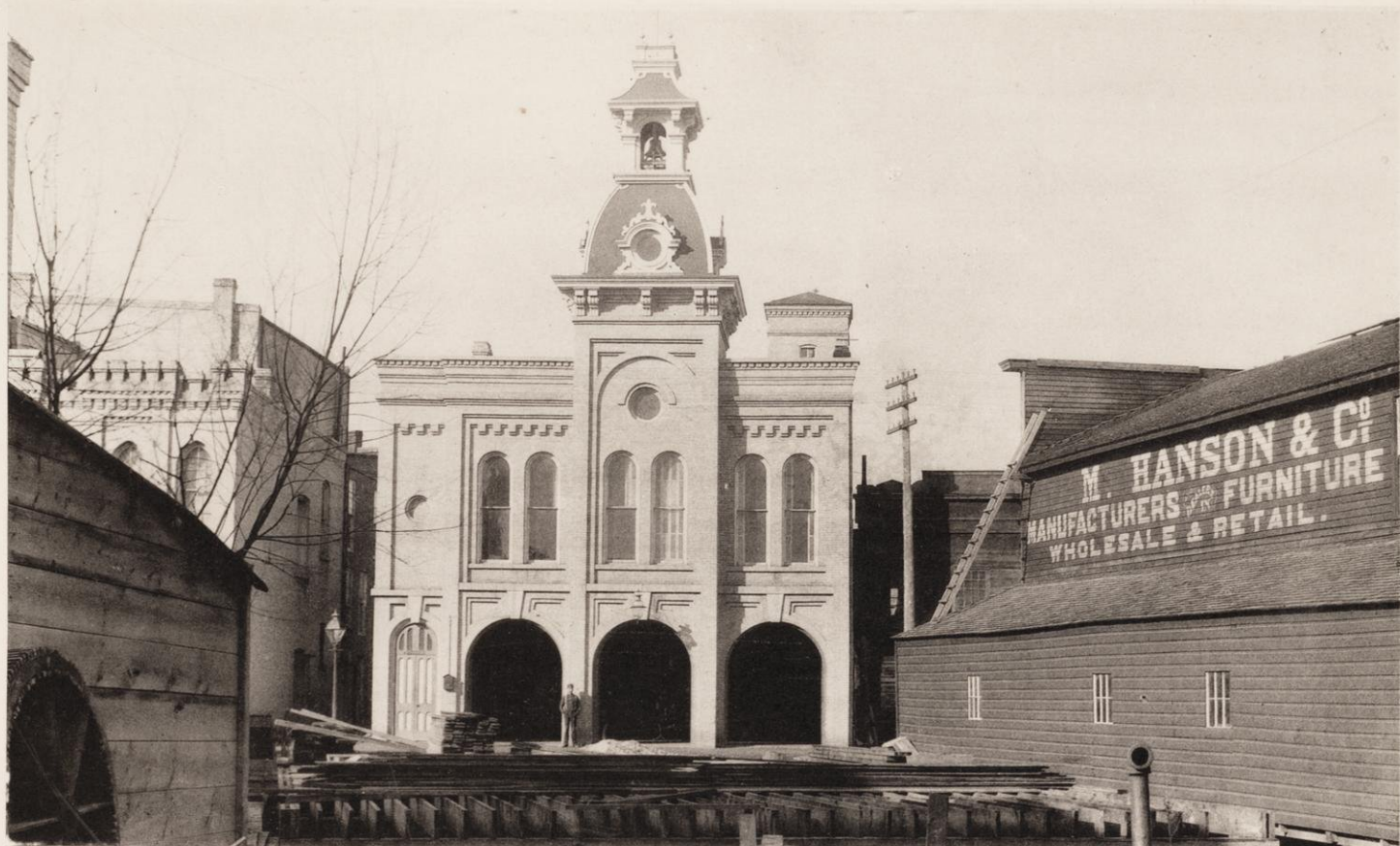
No. 1 Engine House and Council Chamber.
