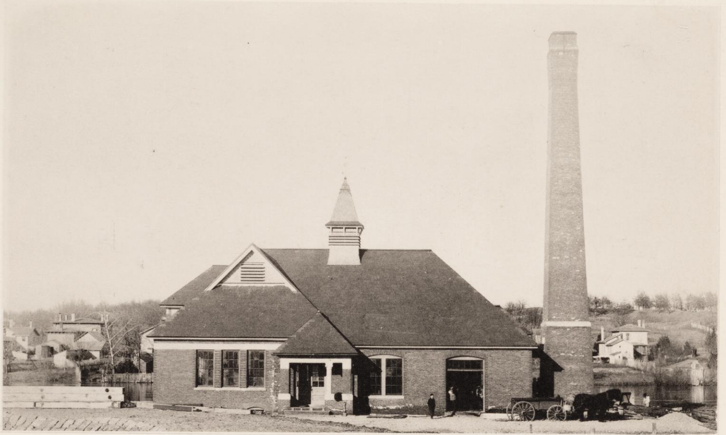
Engine House, Janesville Water Works.
